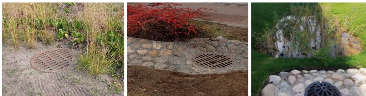
Fig. 8. Emergency overflow directed to the storm water drainage system.
