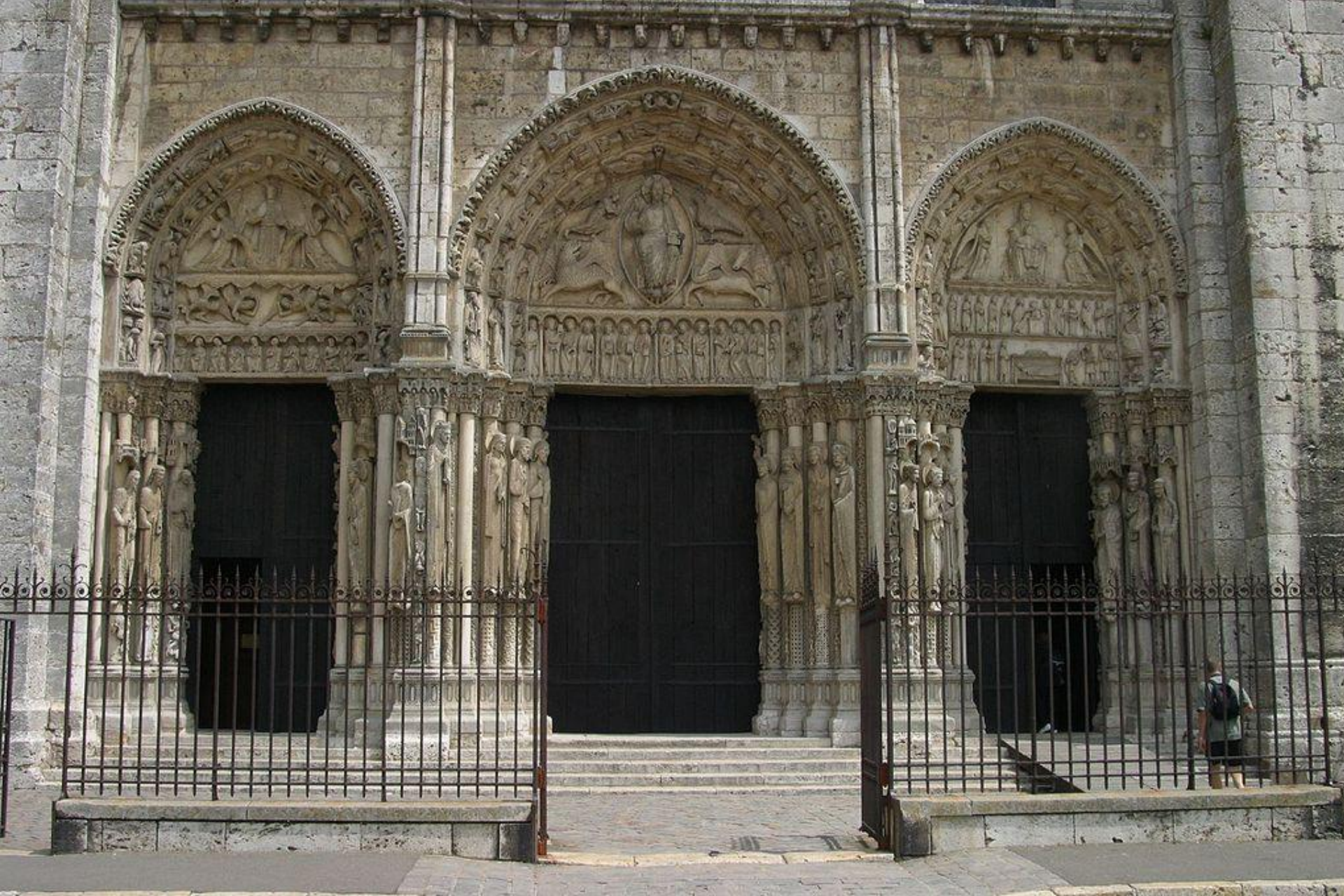
The west façade ( Portail royal )
