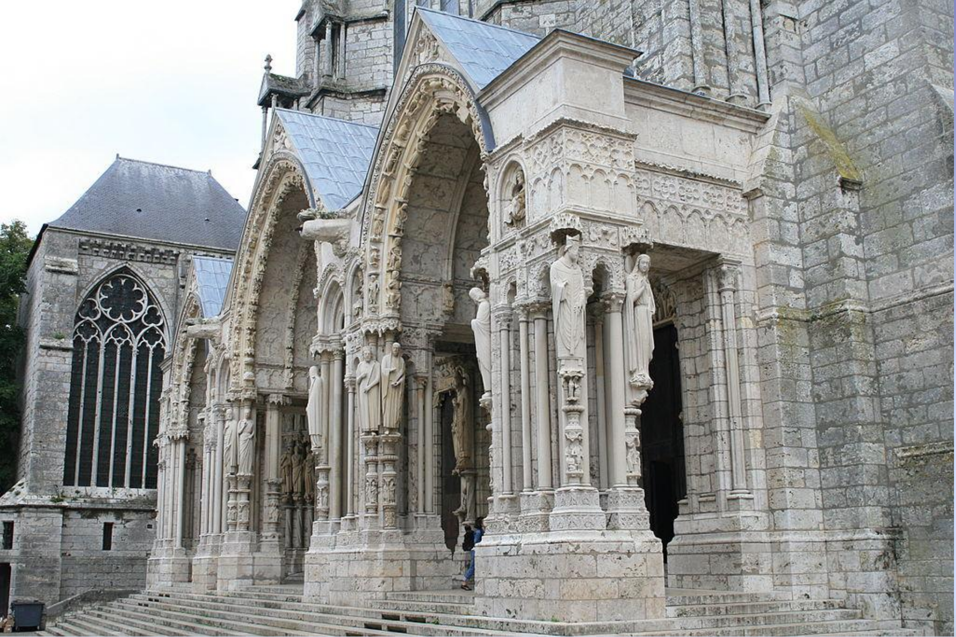
North transept porch with a window of the sacristy (c.1310) in the background
