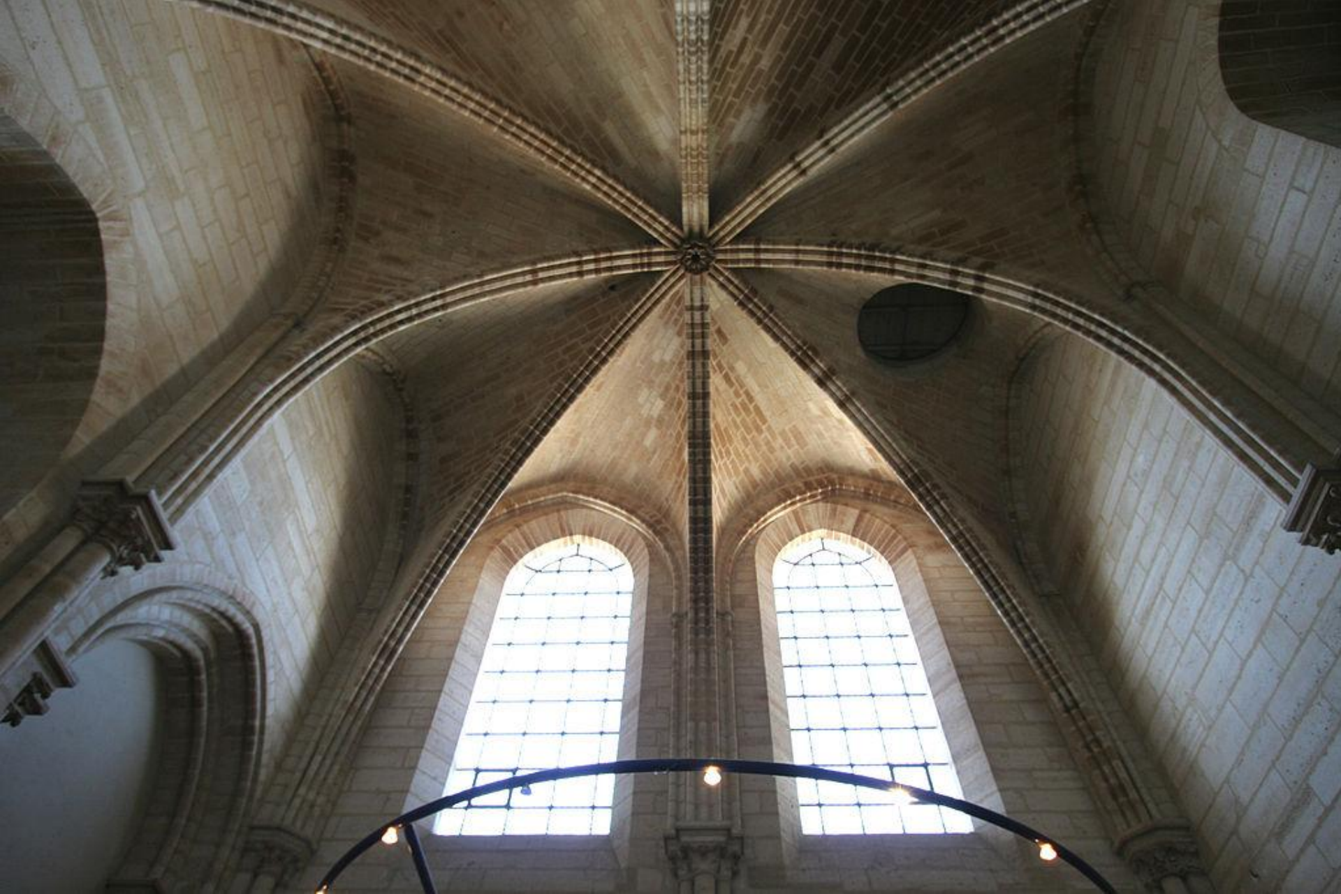
1st floor, room at the North-West, facing the "Parvis"
