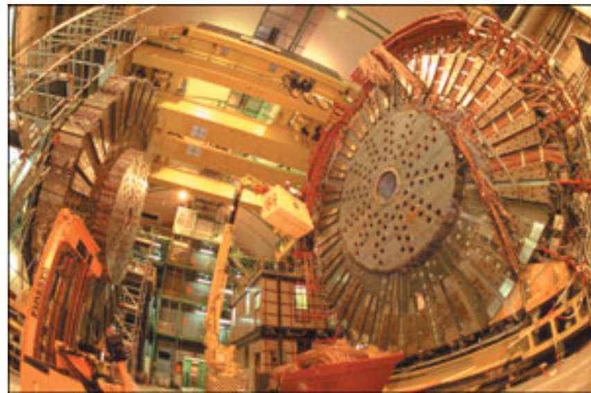
The DELPHI experiment being dismantled at CERN.
